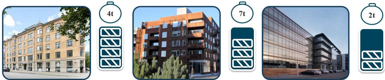
Figure 2: Types of buildings and flexibility in time and energy (4t means 4hours)
