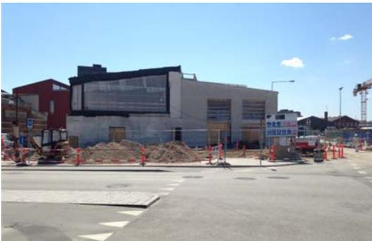
For the demonstration of the recuperation of supermarket waste heat, a *Meny* store (Danish super market chain) has been enrolled and is expected to open at the end of 2018. Planning of the integration of the HOFOR district heating grid and heat recovery of the supermarket refrigeration system is currently in progress. A direct cooperation between Danfoss, *Meny* and refrigeration subcontractor Knudsen Køl has been established.
